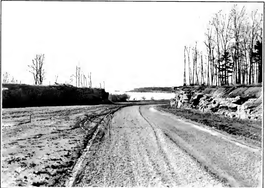
Divided Highway Construction — St. Lawrence River Road, West of Brockville
